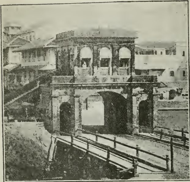
CHURCH GATE, BOMBAY, 1863.
