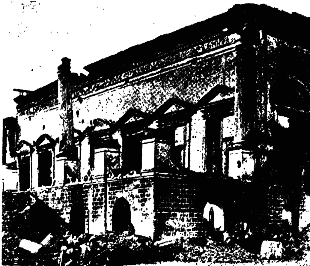
Delhi Bank in Urdu Bazar, Jama Masjid after it was damaged on May 11, 1857.
