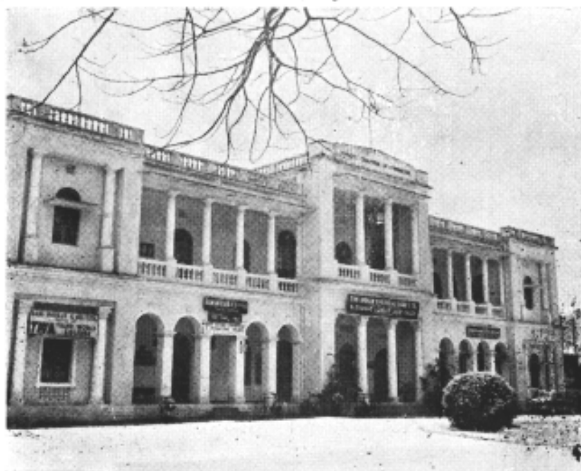
Mysore Chamber of Commerce Building, Kempegowda Road, Bangalore
