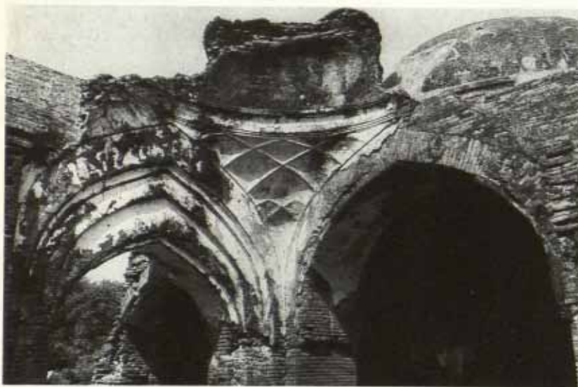
1 Panipat, Kabuli Bagh Masjid, south wing of the prayer-hall, ruined bay with arch-netted pendentives in pseudostructural plaster relief-work. (Photo 1982)
