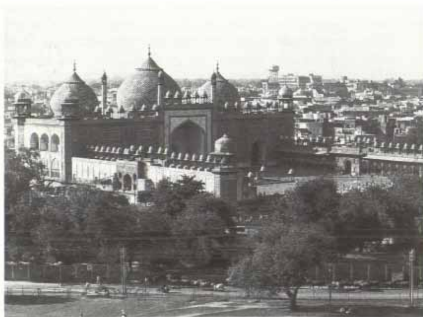
141 Agra, Jami c Masjid, 1058/1648, seen from the Hathī Pol of the fort; the eastern courtyard wing was demolished by the British during the Indian Mutiny in 1857. (Photo 1979)
