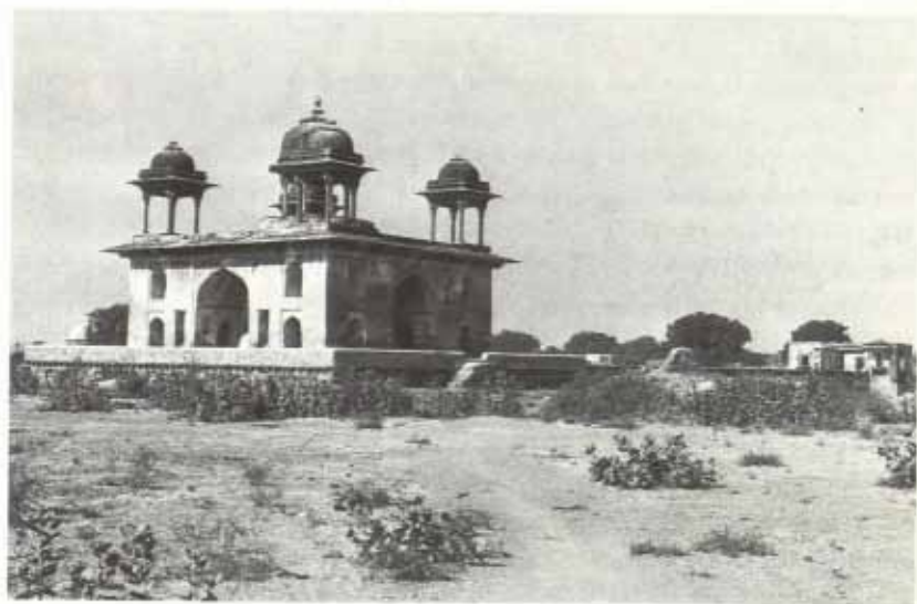
25 Narnaul, water palace of Shah Quli Khan, standing in what used to be an artificial lake, 999-1001/1590-93. (Photo 1979)
