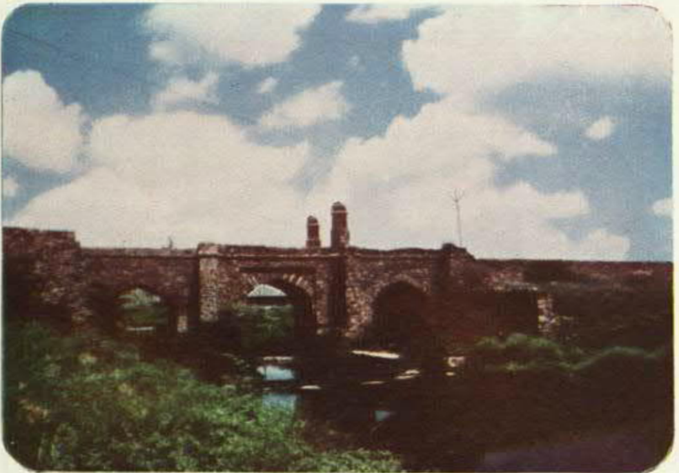
XVT. Khawaja Sarai : Mughal bridge over Budhiawala Nala
