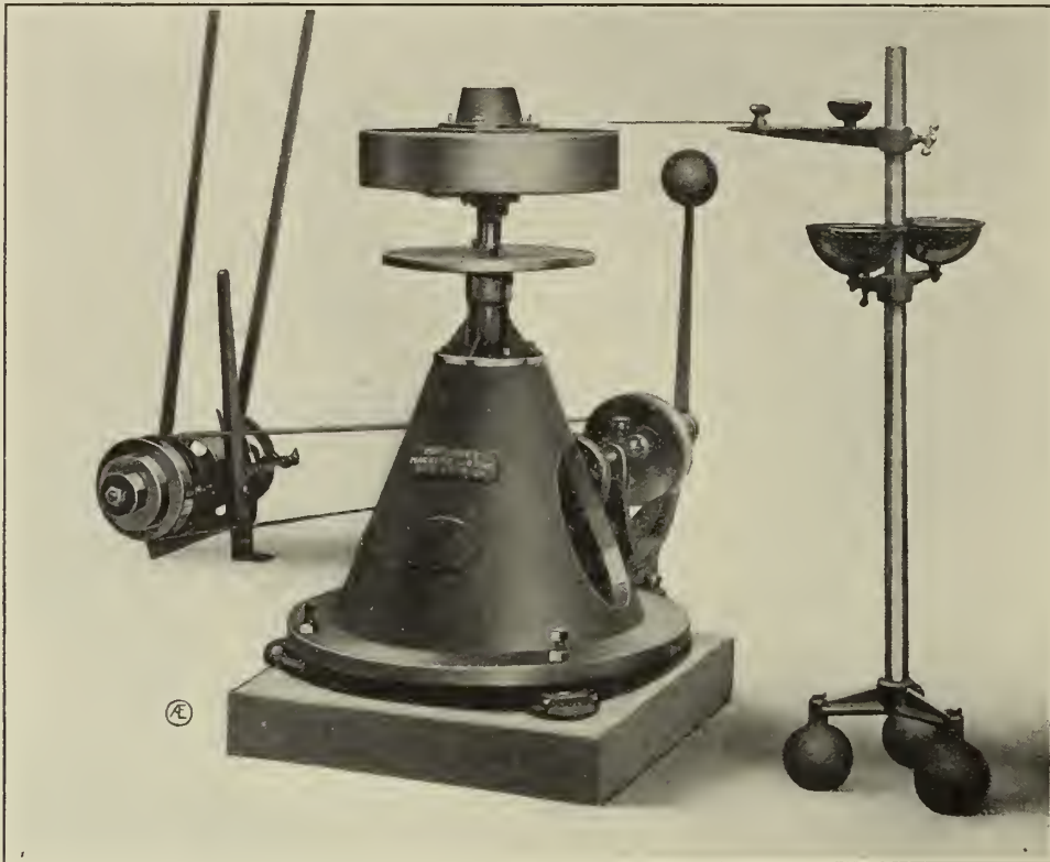
The Defiance Rotational Balancing Machine.
