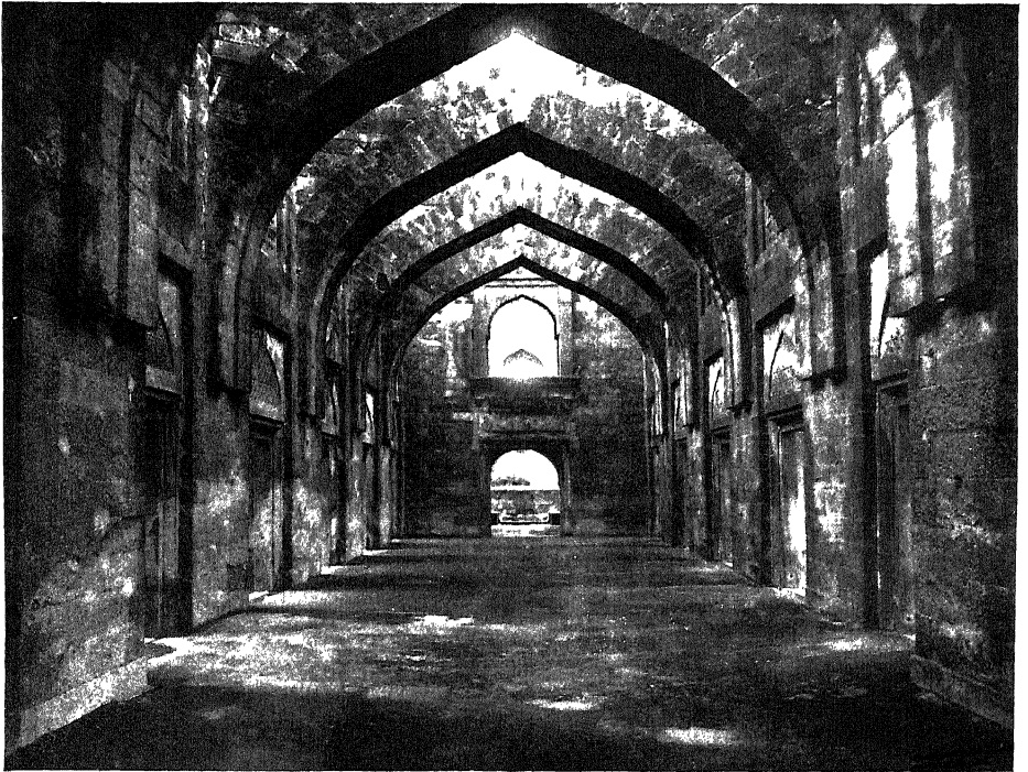
Interior, showing roofless arches
