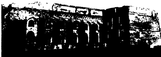
General view from north-east
