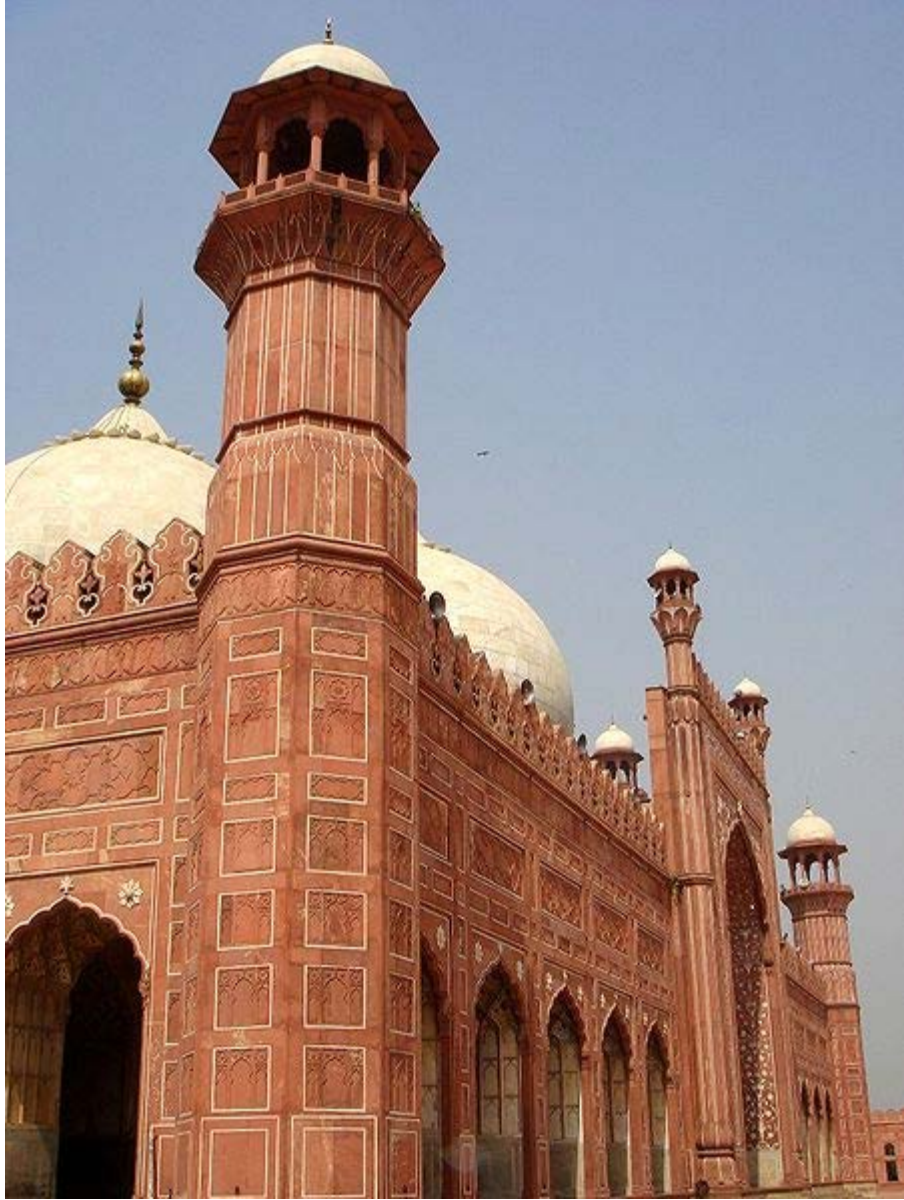
View towards north-west
