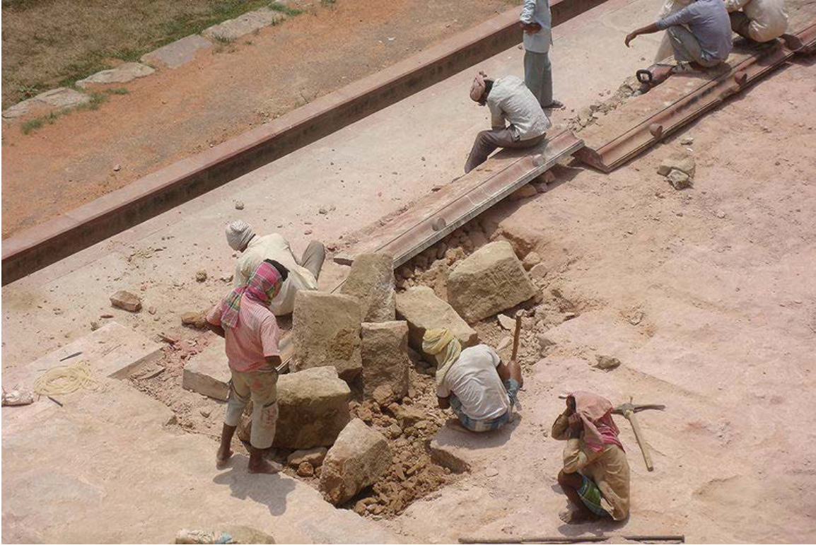
The re-setting and alignment of over 3,000 km of path edging, required some 60 stonecutters, and 2,000 meters of hand-dressed red sandstone slabs that edge the channels (2009)
