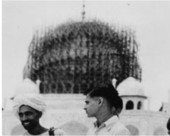
Protective wartime scaffolding
