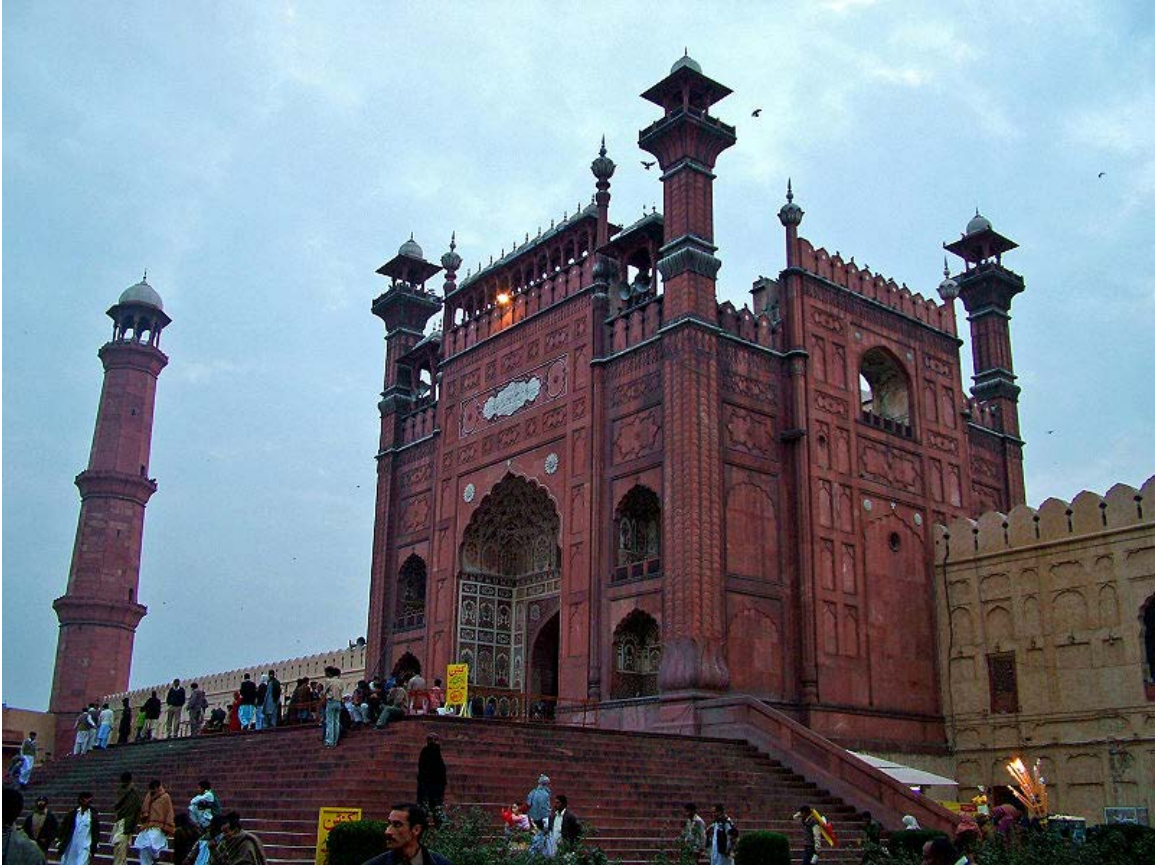
Mosque's main gateway entrance
