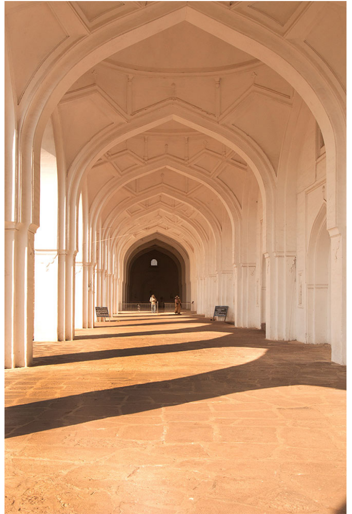
Arch & pendentive detail inside the south liwan.
