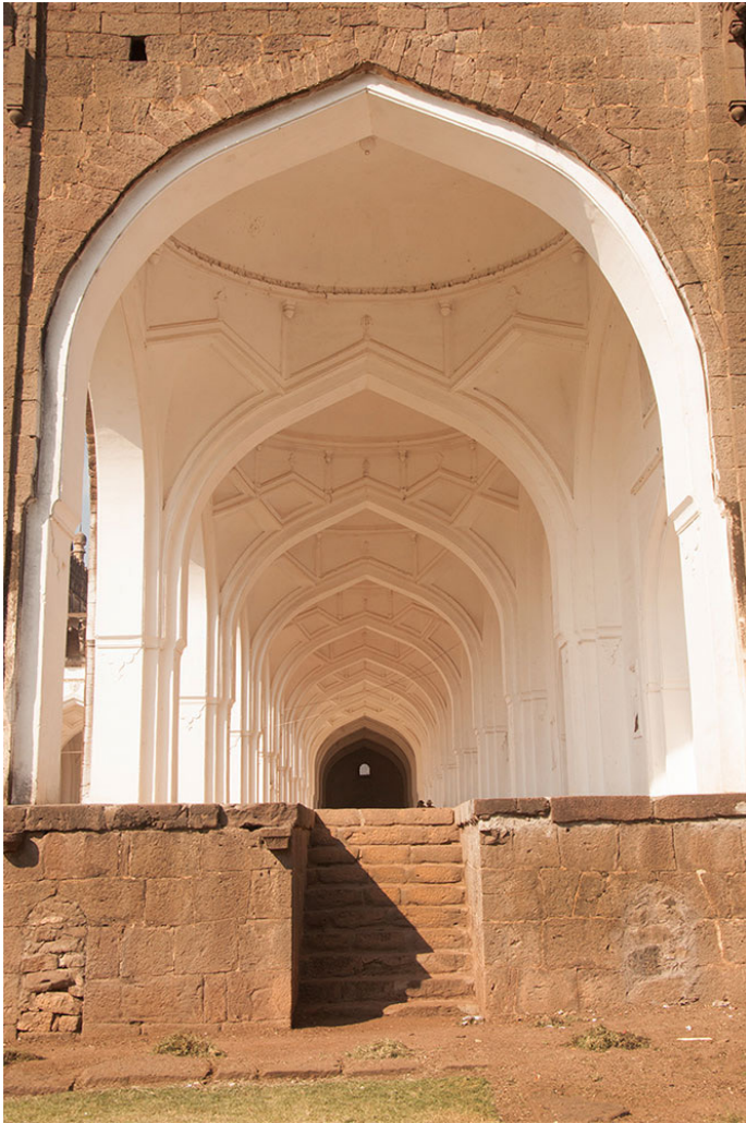
The arch & pendent details.
