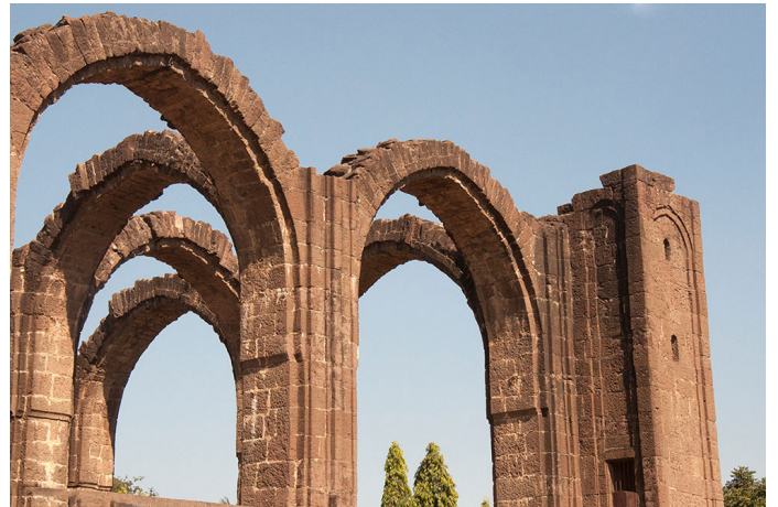
Arches are purely Gothic in outline, being struck from two centers with the curves continued up to the crown.
