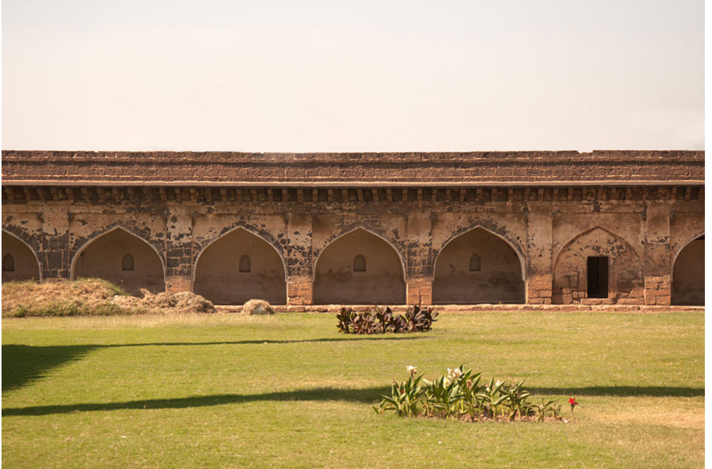
Basement of the mosque.
