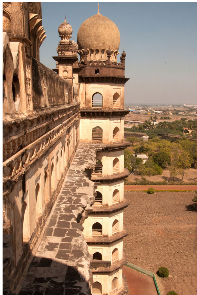
A view from the seventh floor.
