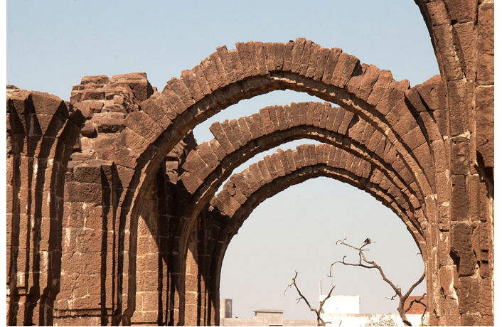
Concentric arch view from inside Bara Kaman.
