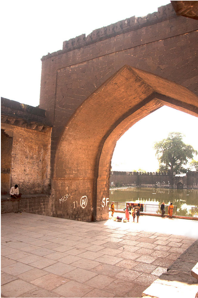
The entrance arch.
