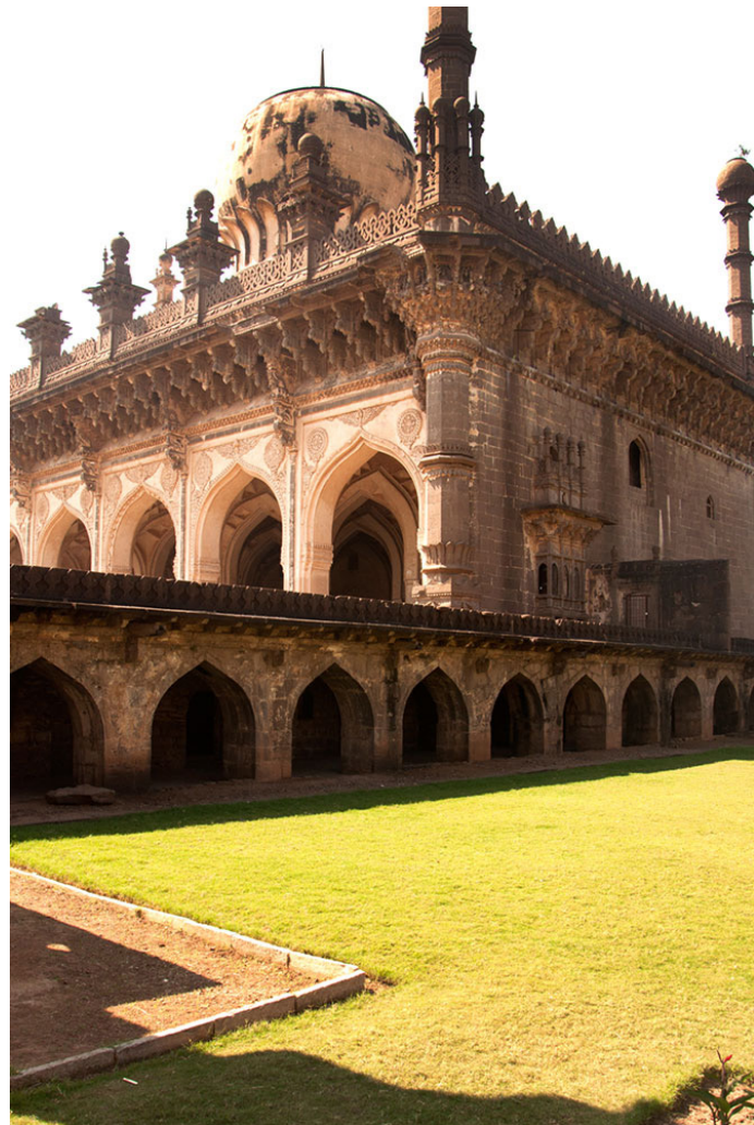
Basement of the mosque.
