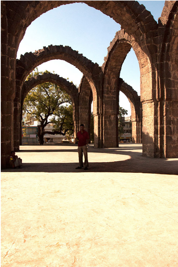
Inside Bara Kaman (12 Arches) is the unfinished mausoleum of Ali Adil Shah II.
