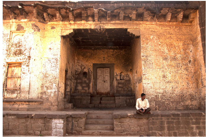
Traveler's room built near entrance.
