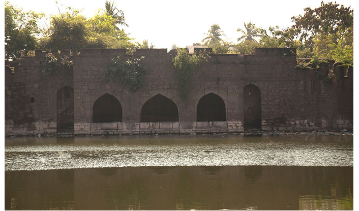
Traveler's rooms with lancet shaped windows.
