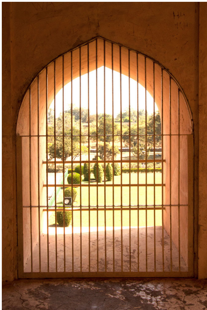
Arched openings at each floor of Winding Staircase.
