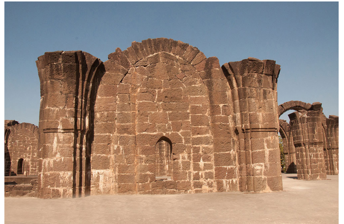
The architect Malik Sandal, initially raised solid walls in the form of concentric arches and once the entire wall was erected, the inner arches were toppled off and only the outermost arch was left intact.
