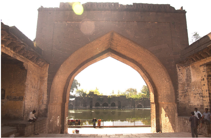
Taj Bawdi constructed in 1620, is one of the interesting sights in Bijapur. Ruler Ibrahim Adil Shah built this well in honor of his queen Taj Sultana. It measures 223 sq feet and 52 feet deep. The entrance to the well has a 35 feet span majestic arch.
