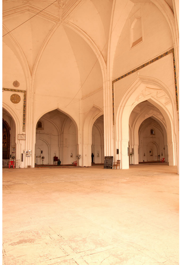
The interior of the sanctuary is a large hall 208' X 107', divided into five aisles by arches on large masonry piers.
