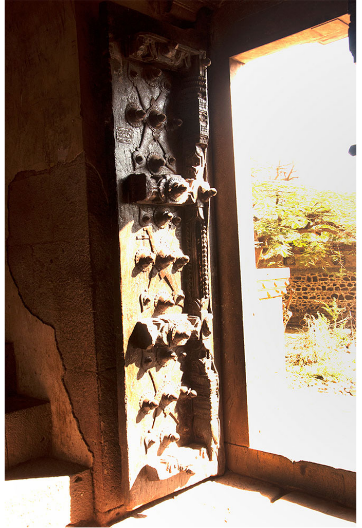
A small side wooden door on the North.
