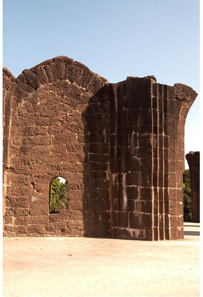
Solid wall in inside Bara Kaman.
