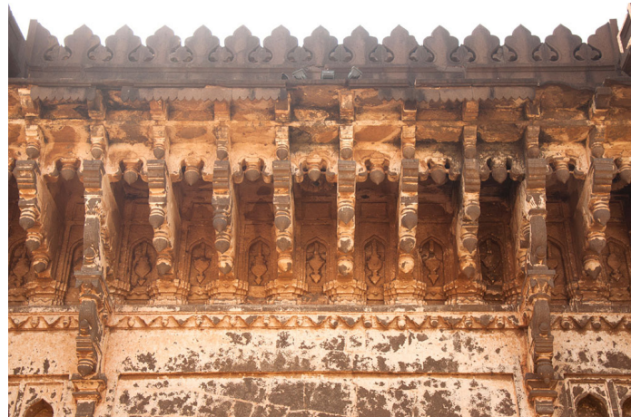
Overhanging and decorative roof.
