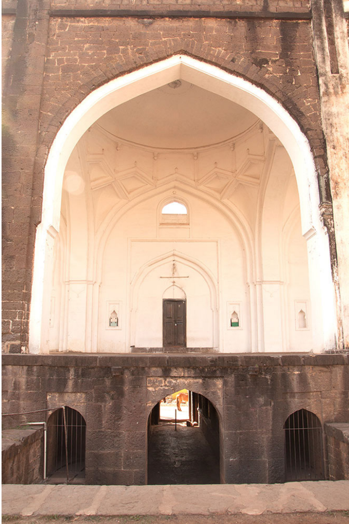
The arches intersect at the top to form an octagonal cornice for supporting the base of the dome.
