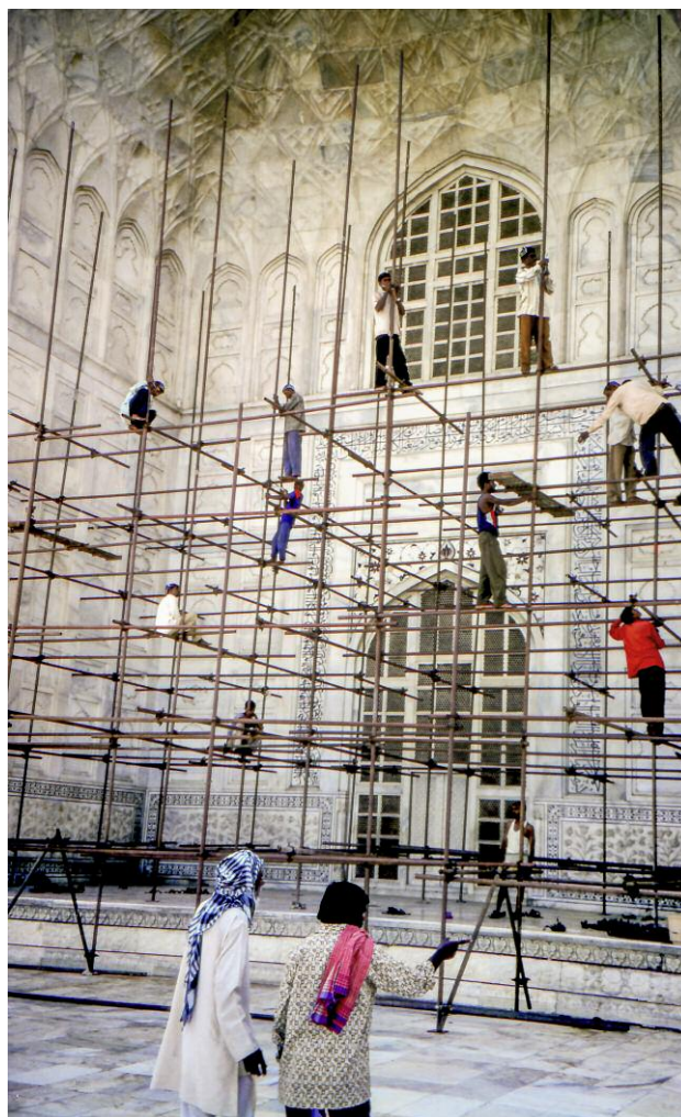
Figure 23. Scaffolding was erected for chemical cleaning of the northern pishtaq of the mausoleum in September 2002. Reproduced with permission of Ebba Koch, 2006.
