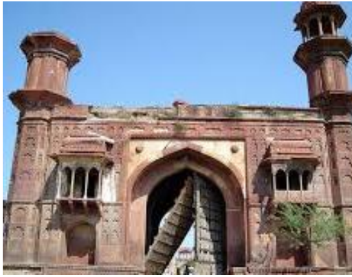
A Caravan Sarai at Jajau, 3kms South of Agra on the Road to the Deccan
