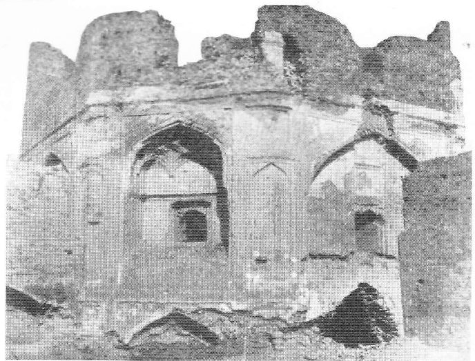
Hameed , Satgarha, Pl. 4: Tomb of Chakar Khan. An old photograph taken before 1964, half of the building is buried under the debris, ghalib kari work is visible the alcoves of as champhered side ,opening is damaged. Later period merlons partially hide and two minarets of original construction
