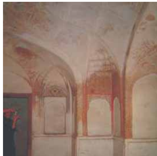
Interior fresco work, Shahi Hammam
