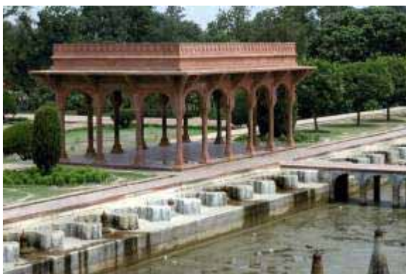
The reconstructed red sandstone Pavillion
