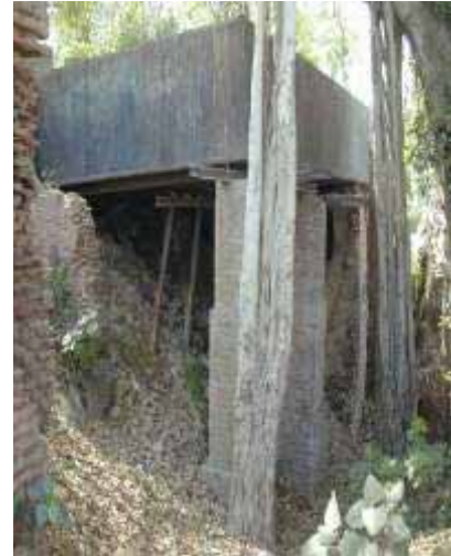
The overhead tank serving the site
