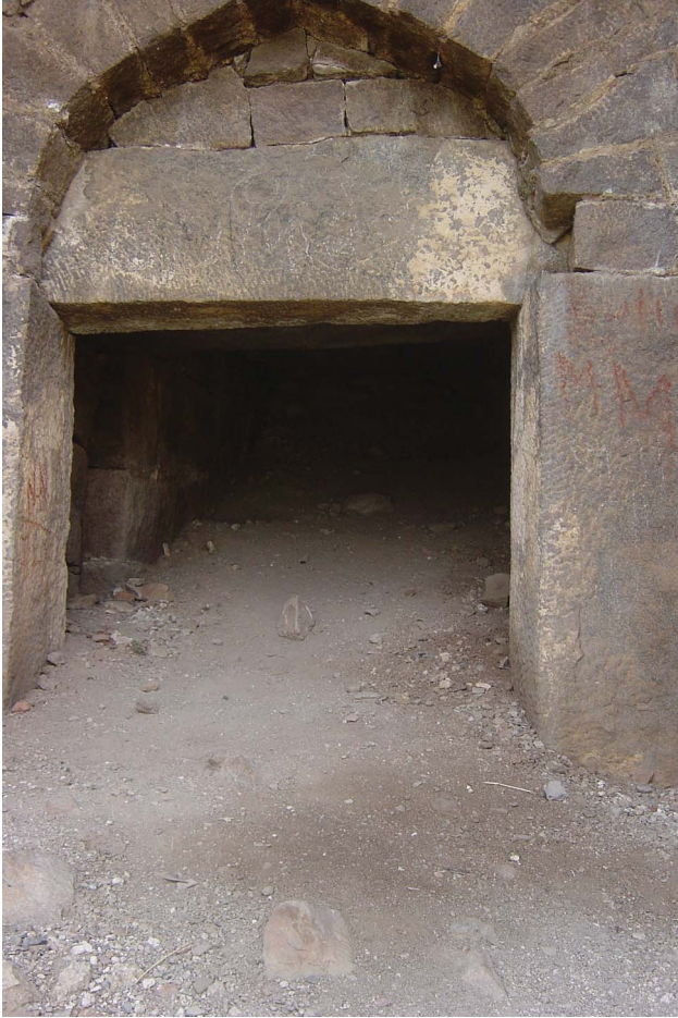
34. Golconda: Bala Hisar walls, second enclosure, door on the north end of the east side, detail.
