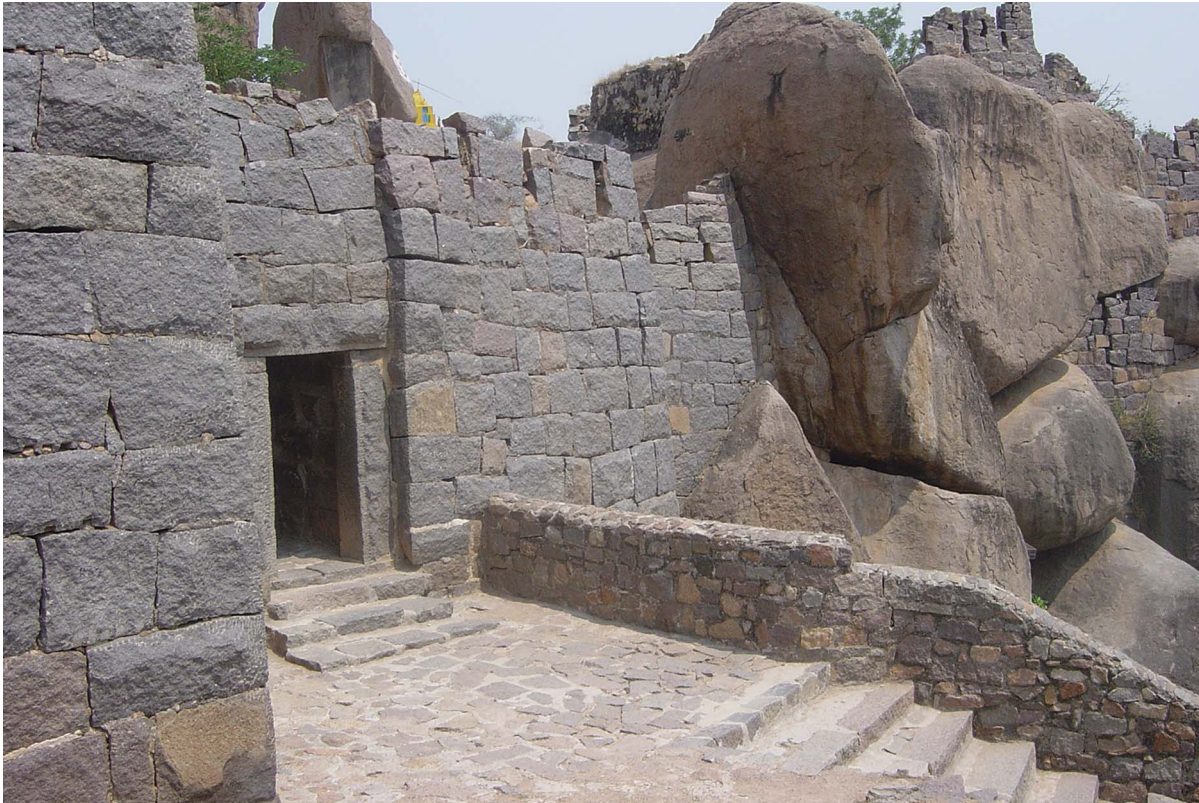
28. Golconda: Bala Hisar walls, first enclosure, south side, door.
