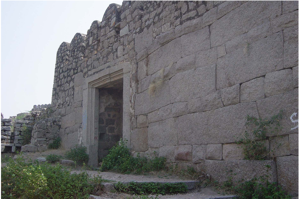
13. Bhongir: doorway and early fortification walls, west side, with alternating courses of headers and stretchers.
