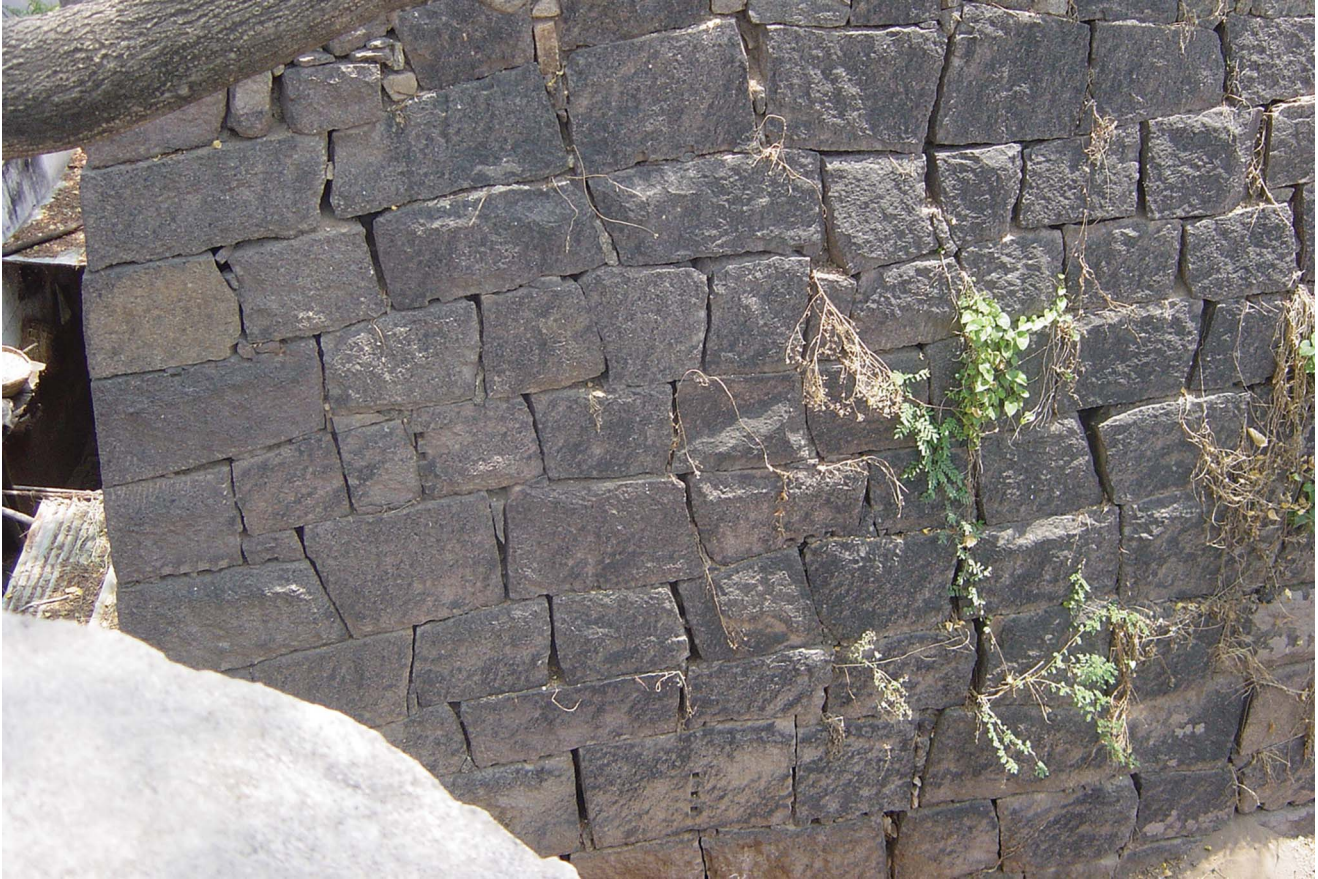
26. Golconda: Bala Hisar walls, third enclosure, north side, passageway preceding gate.
