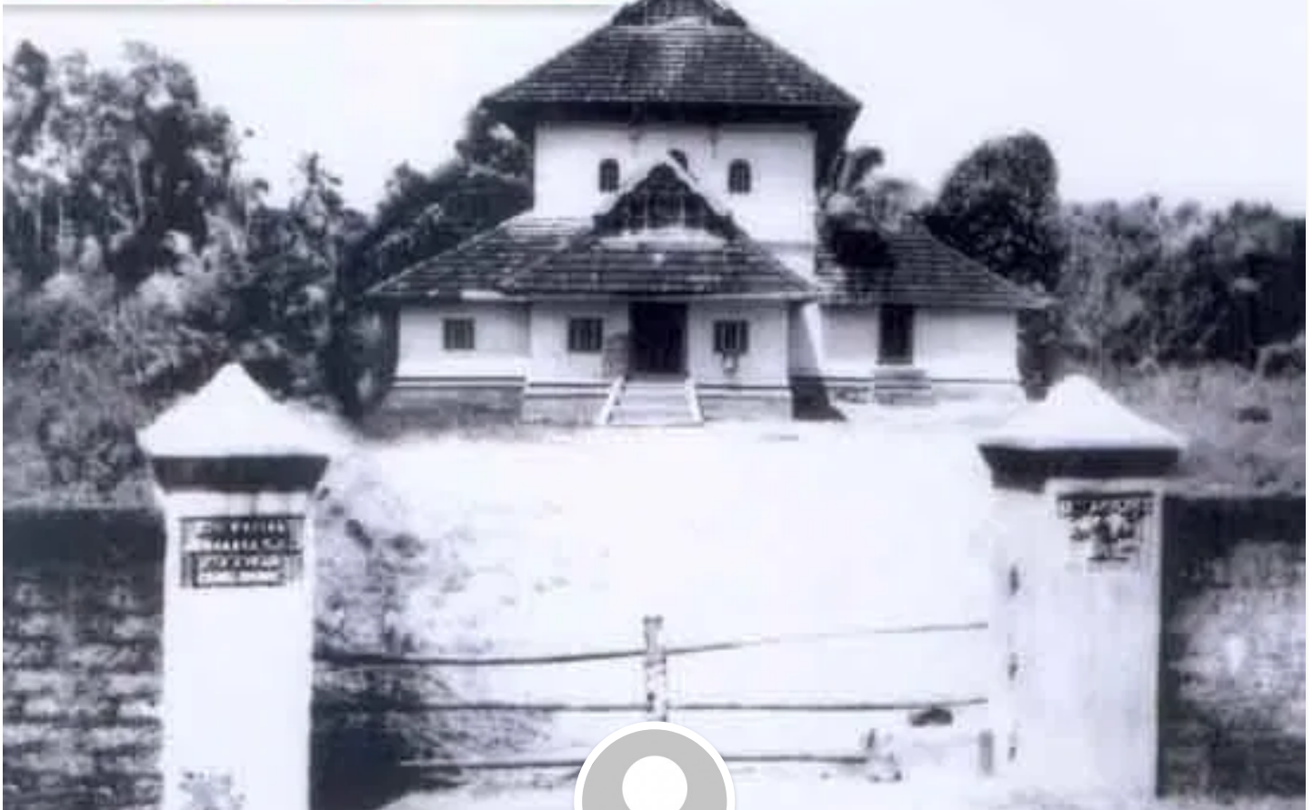
Cheraman Juma Masjid old structure
