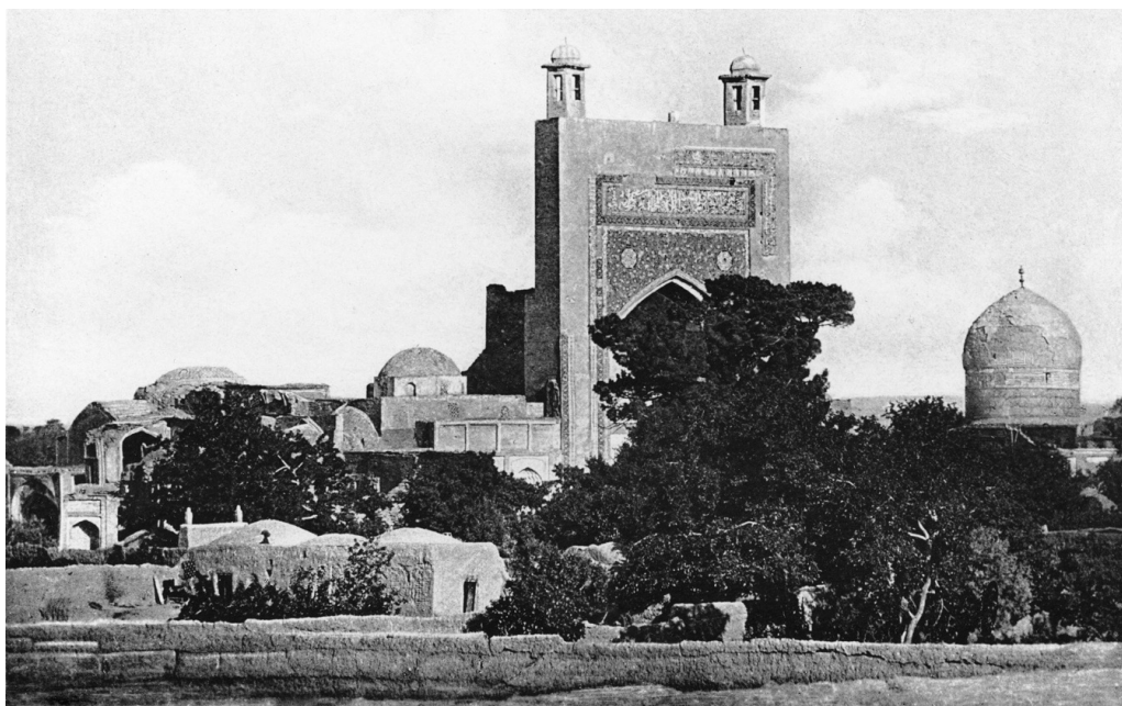
FIGURE 8. Timurid mosque and shrine, Torbat-i Jam, 1913. (From Ernst Diez, Churasanische Baudenkmäler [Berlin: D. Reimer, 1918])
